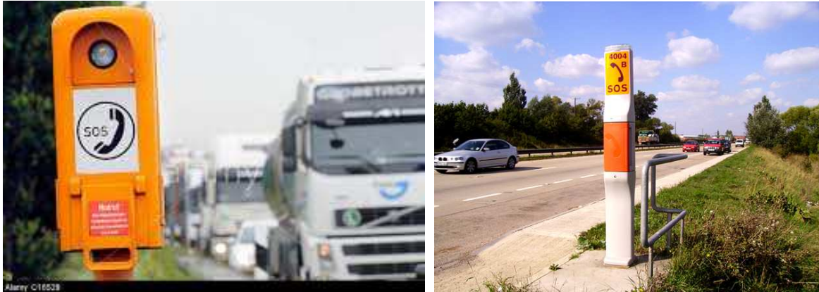
Figure 36. Roadside emergency telephone
